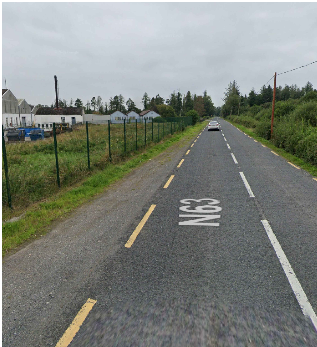
VIEW TO RIGHT OF ENTRANCE (West)
